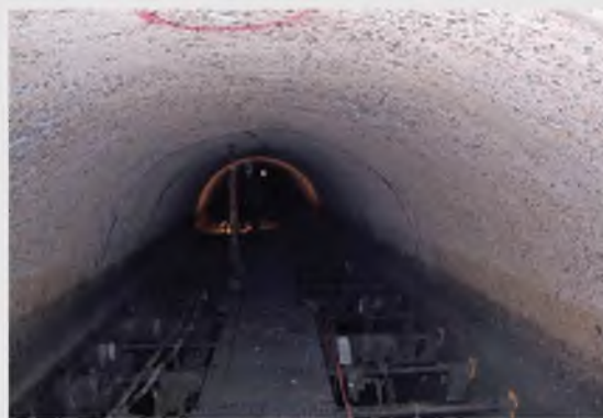
Inside of pipe pressure-washed in first 8-hour closure. Note the very rough surface with exposed aggregate caused by cement paste loss.
