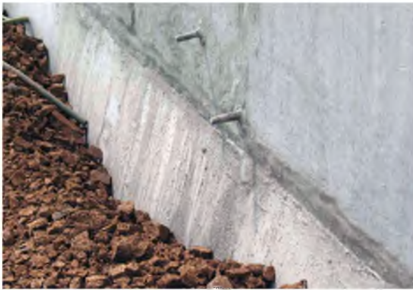
Capped area with Xypex injection ports installed
