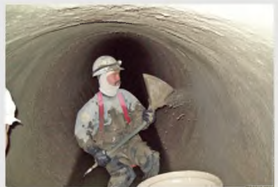
Xypex Concentrate followed by Xypex Megamix I is applied in second 8-hour closure.
